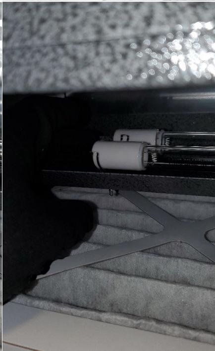
On the other end, push the lamp into the clip to secure it.
